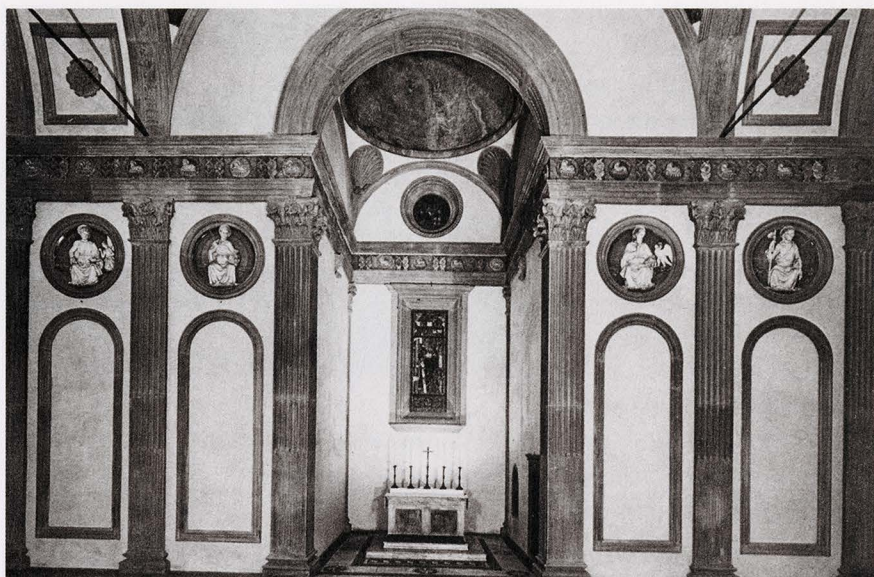
Figure 8: Pazzi Chapel, Florence (1429-1433, Filippo Brunelleschi [1377-1446]). Interior view illustrating diffuse lighting.
