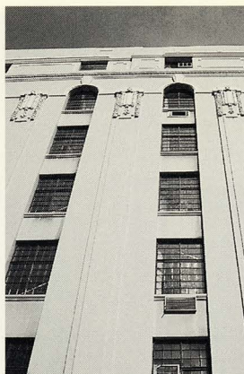
19 Grant, Jackson's Warehouse & Showrooms (now the SA Perm), 1930
