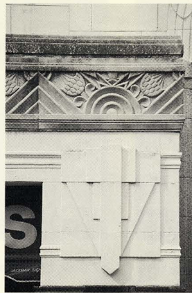
29 Grant, Commercial Union Building, detail of façade mouldings, 1932
