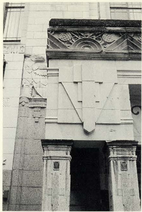
27 Grant, Commercial Union Building, detail of terrazzo colonnade, 1932
