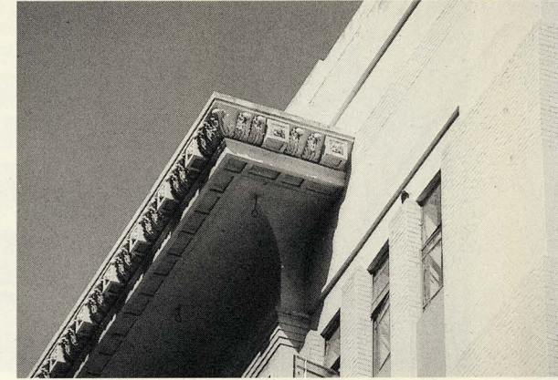
16 Grant, Boston House, detail of acanthus moulding on cornice, 1929
