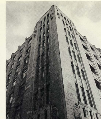
26 Grant, Commercial Union Building (now Market House), 1932
