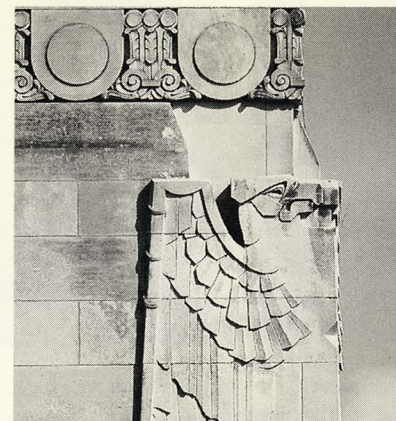
31 J A Wetmore, Main Post Office, Kansas City, detail of façade, 1933-1935
