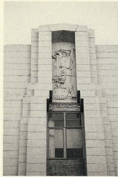
33 Quail, Versorging, pre-cast concrete panel, 1932
